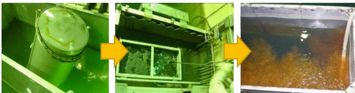
Fig. 1. The Decontamination of the Spent IERs in Tank of the Spent Fuel Pool.
